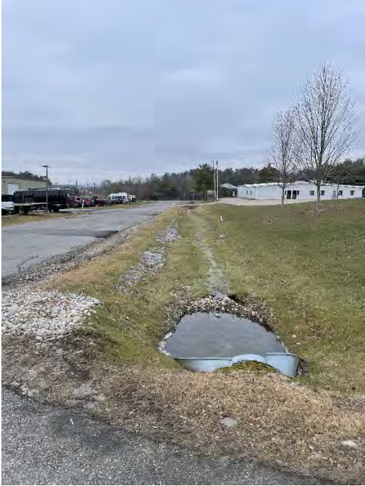
Figure 1: Looking northbound along Wilson Rd. STP to be located in swale.
